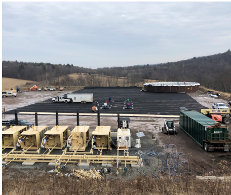
Drilling and Completion Pads
