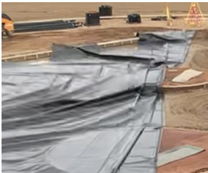
Liner deployment during rain window.
