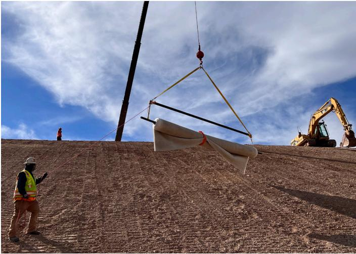
Crane behind berm, using spotter to place RCR® material.
