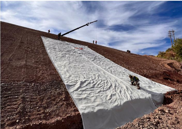
RCR® overlap and seaming. Bottom of berm anchor trench placement.
