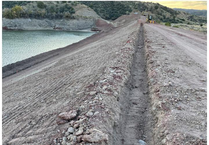
Site prep with top of berm anchor trench placement.
