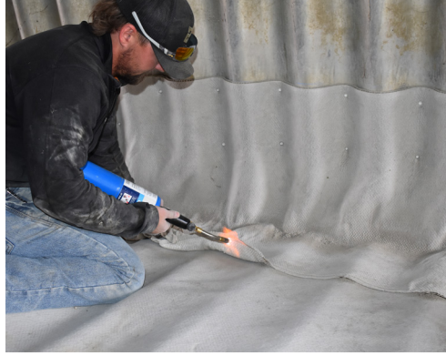
Heat welding RCR® seams
