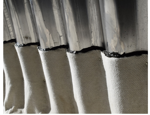
Wall panels secured and sealed
