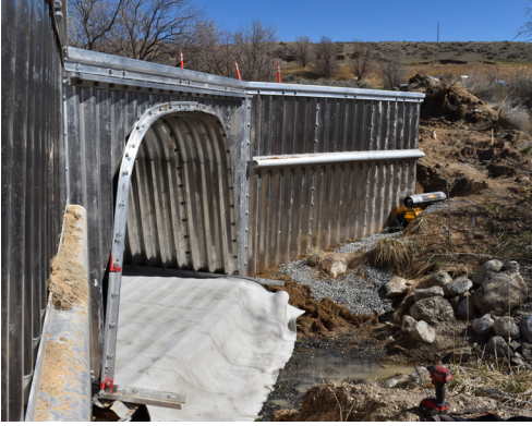
RCR lining outlet to fish run/wildlife habitat
