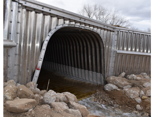
Addition of riprap to enhance erosion control
