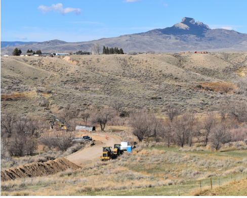
Remotely located culvert in Cody, WY
