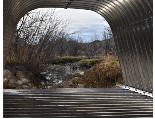
Culvert before remediation
