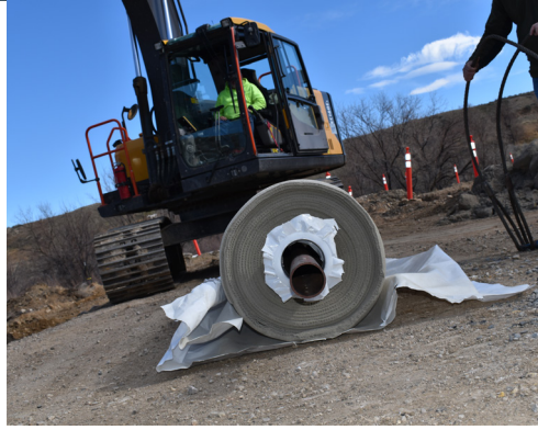
Unloading & prepping RCR®
