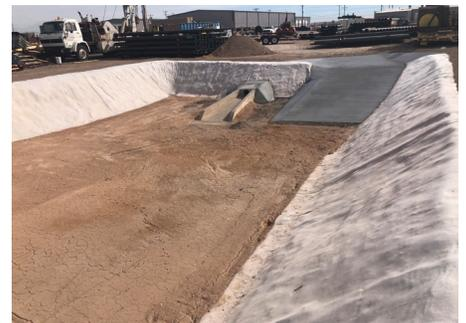
**THREE DAY INSTALLATION** *Day One:* Grading and trenching performed utilizing 2' down 1' back at the top and bottom of the slope. *Day Two:* 75% of material was deployed for the facing slopes. *Day Three:* remaining 25% of material installed and entire project hydrated using water truck with pump. Comparatively, a local contractor estimated the project would take 1-2 weeks if traditional concrete methods were utilized.
