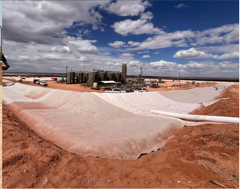
RCR® installation to redirect water runoff and prevent further erosion.
