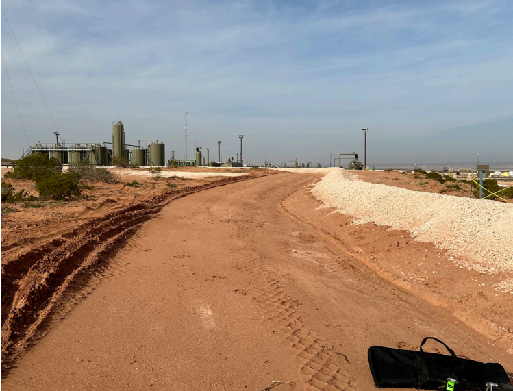
Compacted subgrade preparation prior to RCR® Installation
