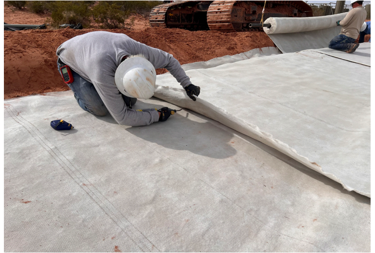
Seam welding with handheld heat torch
