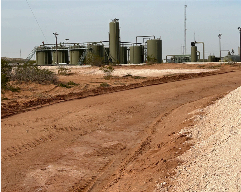
Ground work preparation prior to RCR® Installation
